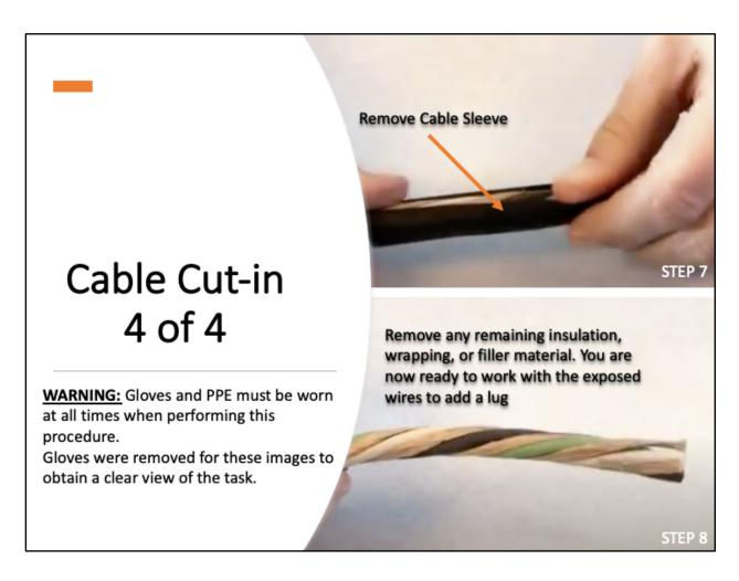
Carefully separate the sleeve at the lengthwise cut and remove it from the conductor. Remove any remaining insulation, wrapper, and filler to expose the bare conductor.
