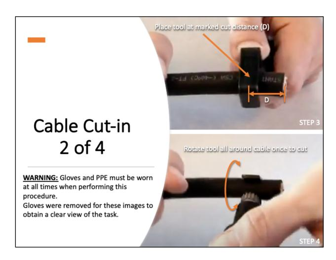
Place the cutting tool perpendicular to the cable at the previously marked location for insulation removal and then rotate the cutting blade all the way around the cable.
