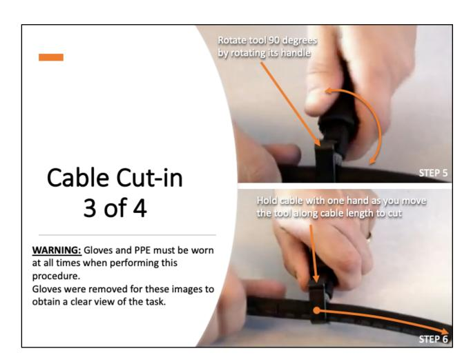
After you have cut all the way around the insulation, rotate the cutting blade and cut the sleeve lengthwise to the end of the cable.
